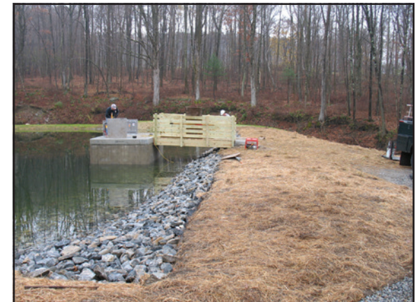
Newly constructed dam improvements
